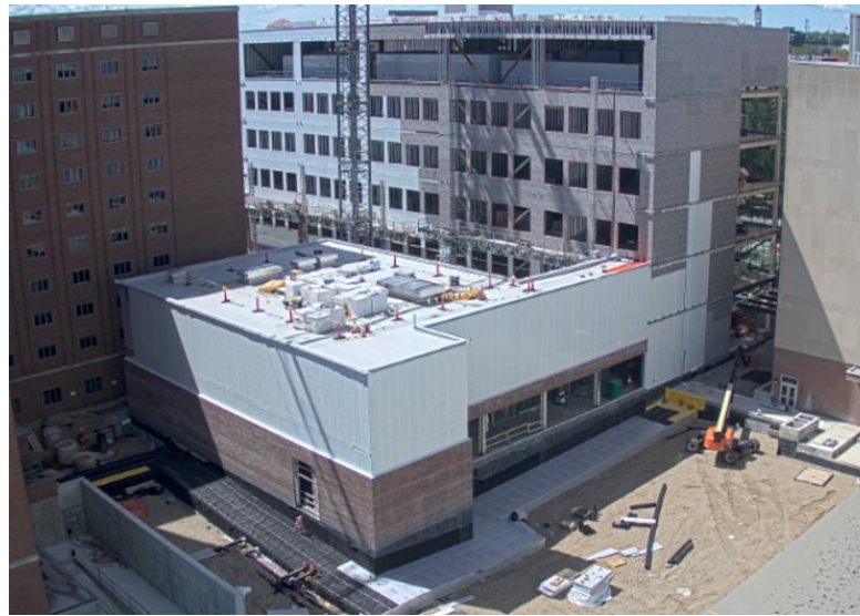
Progress as of December 2025
